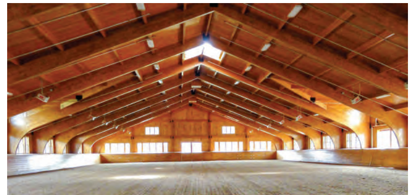
GLUE-LAMINATED ARCH ARENAS
